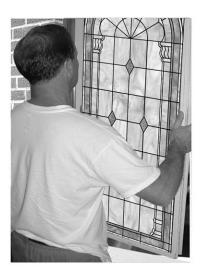
4. Using helpers on both sides of the window carefully set your window into place. Shim and level window until it is stable
