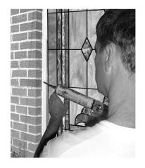
Apply polyurethane caulk to the outside of the window between brick and frame to weatherproof wiping off any excess caulk.
