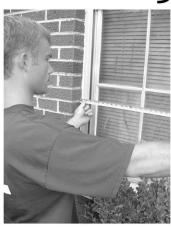
1. Before ordering your windows, measure your window opening carefully, taking the distance from brick to brick and subtracting 1/2" from both width & height to ensure proper fit.
